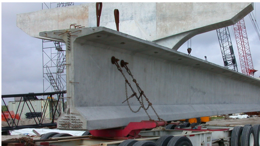
Figure 2.12 Chain braces on Florida Bulb-Tee during transportation
